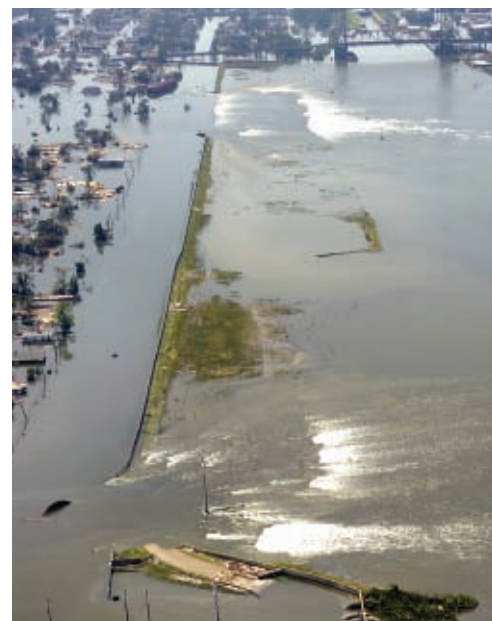
Figure 3 This levee near New Orleans broke as a result of Hurricane Katrina, allowing the Mississippi River through.
